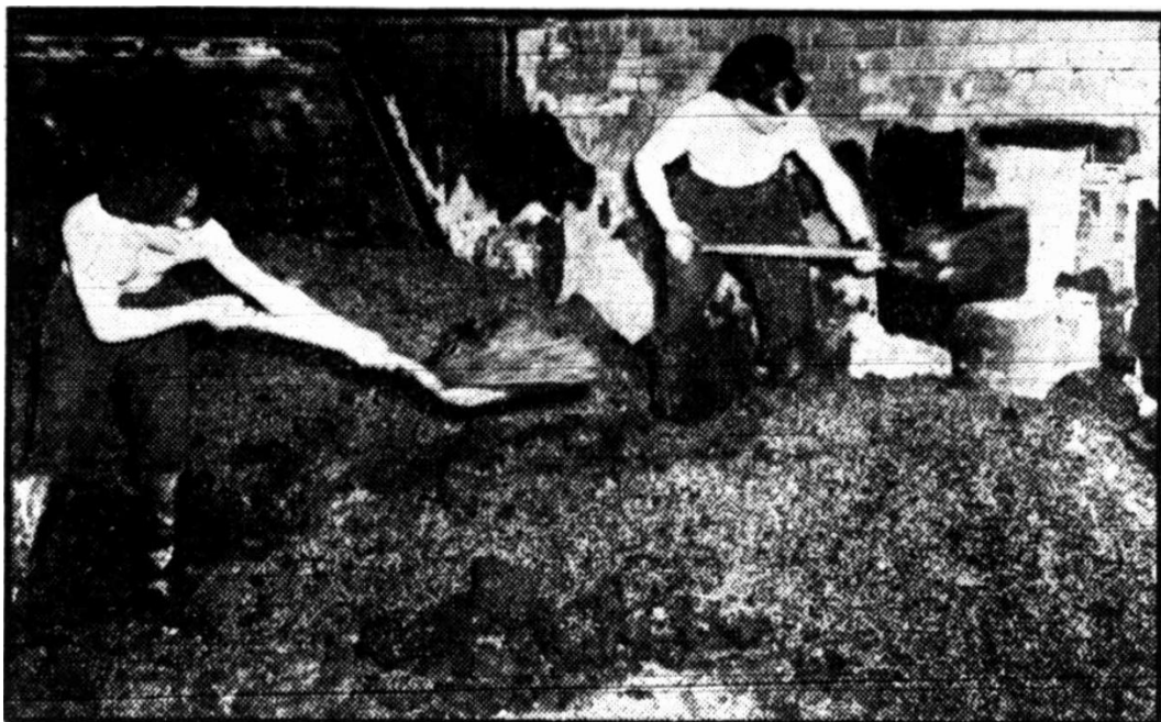
FIREMEN R. Oates and L. Cahalan shovelling burnt barley in one of the roasting ovens at the Lion Brewing and Malting Co., Ltd., Melbourne street, North Adelaide, after a fire early today. Firemen battled for an hour to control 30-ft. flames. (Story-Page 1.)
