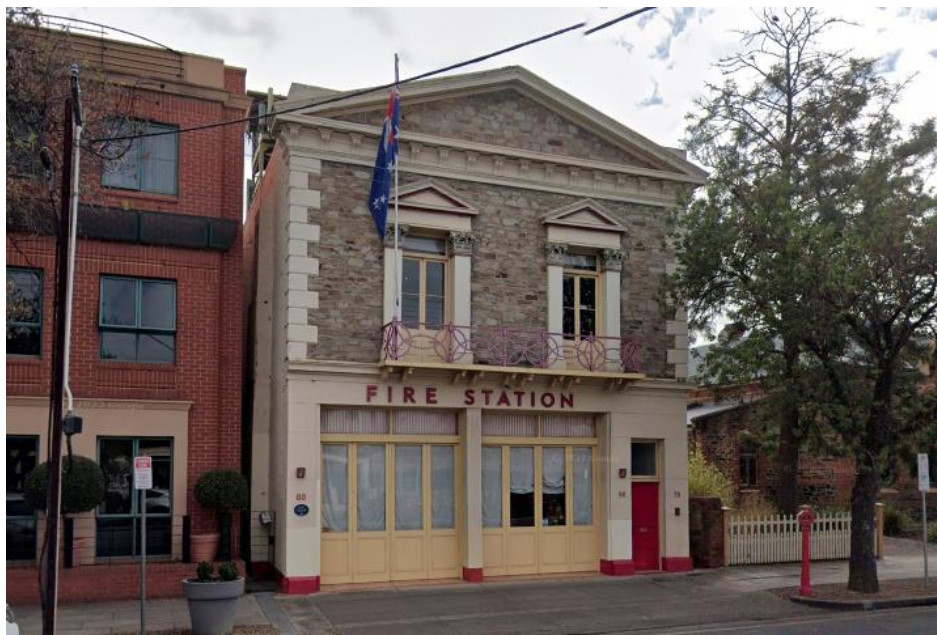
North Adelaide Fire Station 2024 Google Maps
